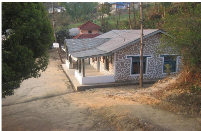
ANCIENT ADMINISTRATIVE BUILDING
